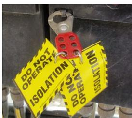
**Figure 10 - Example of multi-hasp for use on an electrical isolation**
